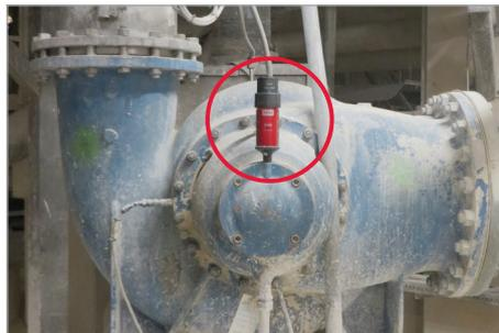
Bearing lubrication on a pump
