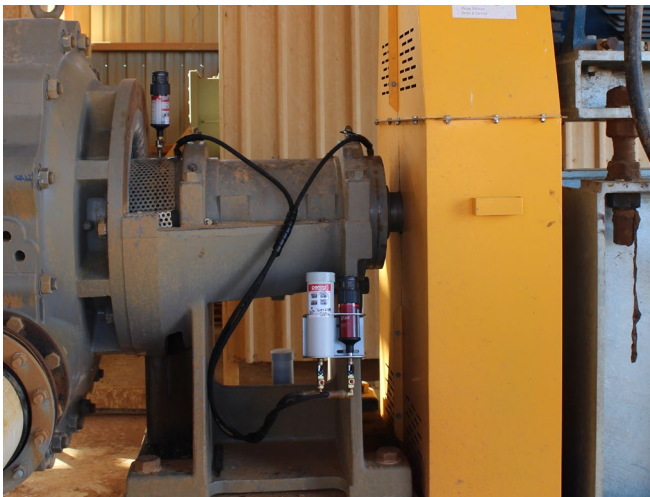
Application Labyrinth seals and mechanical seal Lubricator perma STAR VARIO 250 cm 3 Installation kit K230C & direct mount
