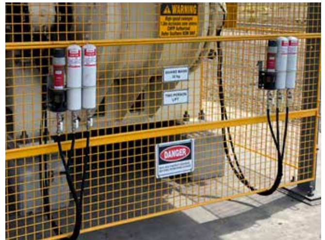
Application Conveyor pulley bearings and seals Lubricator perma STAR VARIO 500 cm³ Installation kit 2 x K3CHCX
