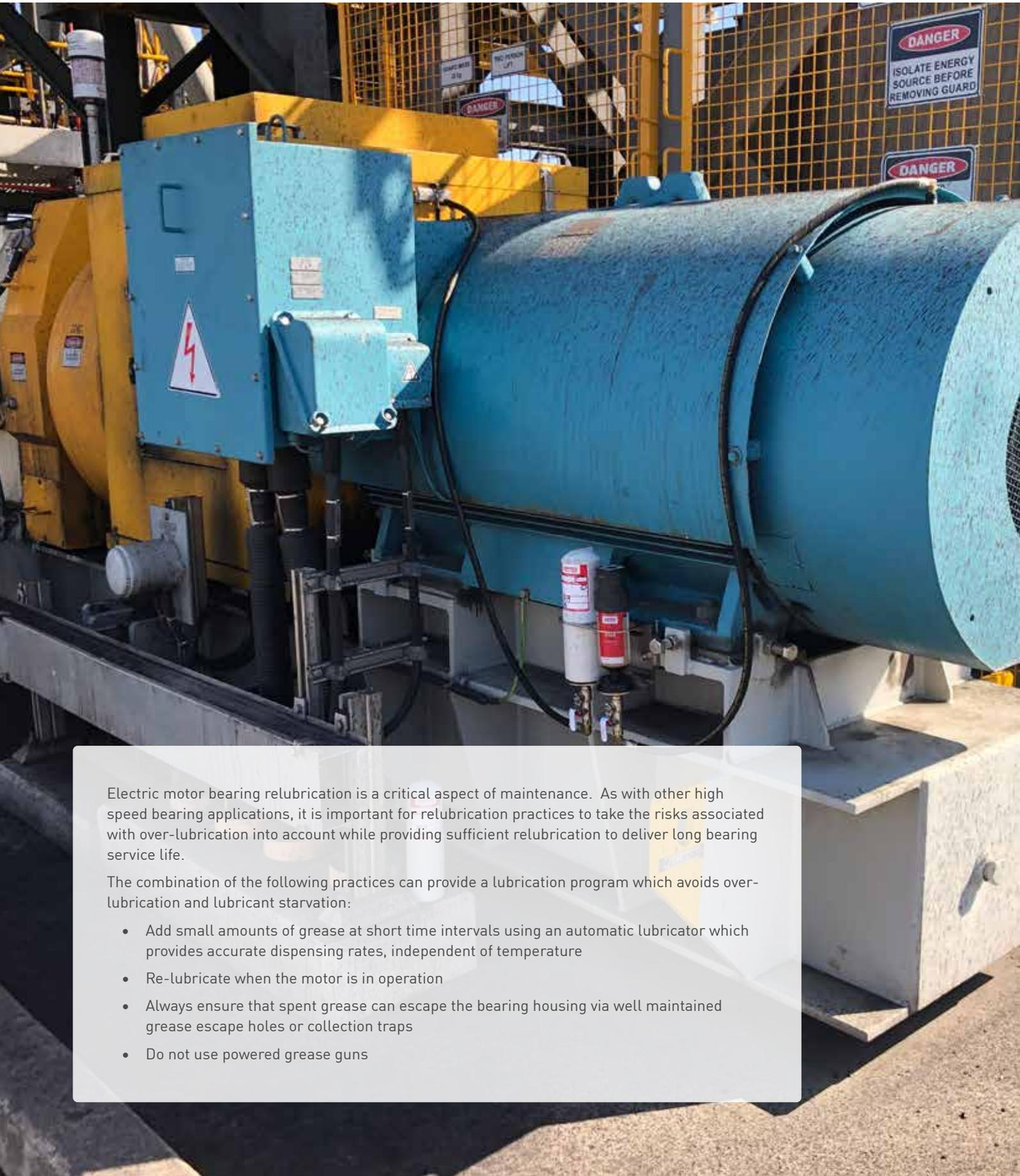
Electric motor bearing relubrication is a critical aspect of maintenance. As with other high speed bearing applications, it is important for relubrication practices to take the risks associated with over-lubrication into account while providing sufficient relubrication to deliver long bearing service life.
