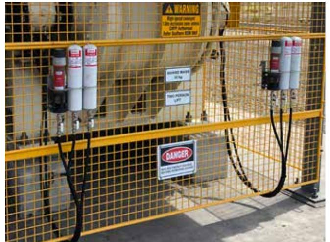
**Application** Conveyor pulley bearings and seals
