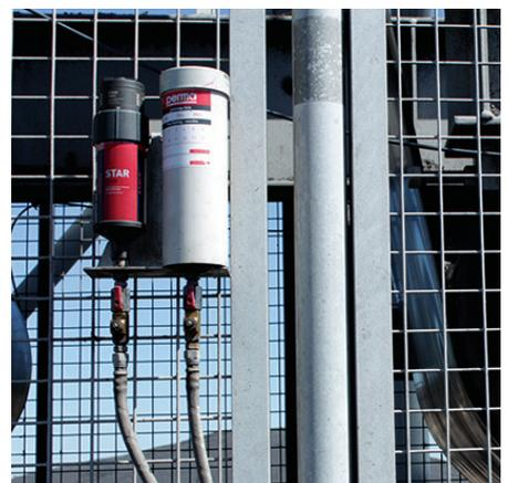
**Strategy 3** – Automatically lubricate equipment which would otherwise require working at heights or confined space permits.
