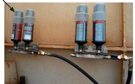
Seal all connection parts with a metal bonding adhesive (medium)
