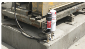
Pump bearings and seals
