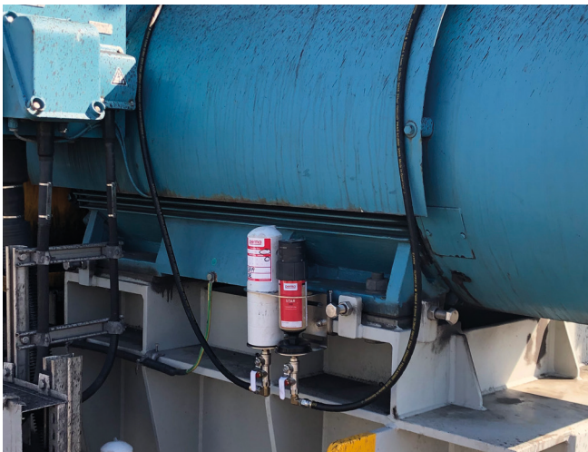
Application Electric motor Lubricator perma STAR VARIO 250 cm³ Installation kit K230C
