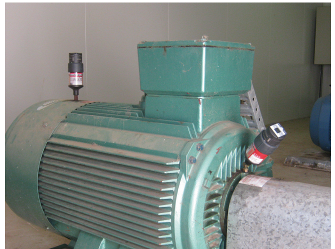
Application Electric motor Lubricator perma STAR VARIO 120 cm³ Installation kit Direct mount
