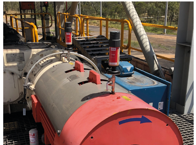
Application Electric motor Lubricator perma STAR VARIO 250 cm³ Installation kit KDSV-708V
