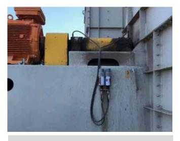
Application Fan support bearings perma STAR VARIO 250cm³ Lubricator Installation kit K230
