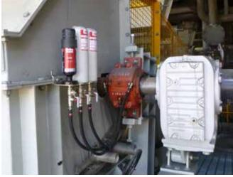
**Application** Conveyor pulley bearing and seal **Lubricator** perma STAR VARIO 250cm<sup>3</sup>
