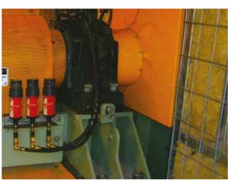
**Application** Fan support bearings Lubricator perma STAR VARIO 250cm³ Installation kit K330
