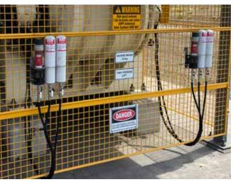
Application Conveyor pulley bearings and seals
