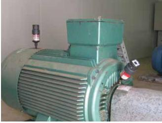
Application Electric motor Lubricator perma STAR VARIO 120cm<sup>3</sup> Installation kit Direct mount
