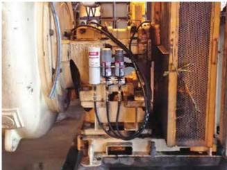
Application Labyrinth seals and gland seal Lubricator perma STAR VARIO 250cm<sup>3</sup>
