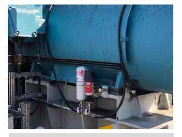
**Application** Electric motor perma STAR VARIO 250cm³ Lubricator
